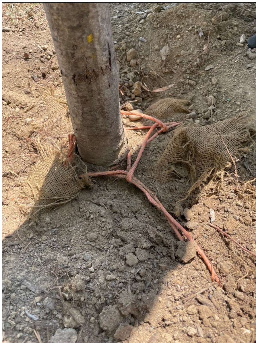
Photograph 17: Per ANSI standards, balled and burlap trees should have twine, burlap and the top 1/3 of the wire basket removed
