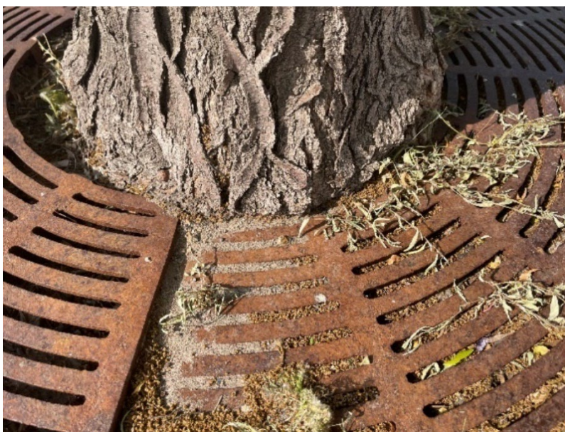
Photograph 6: A grate is girdling a honeylocust street tree stem (trunk).
