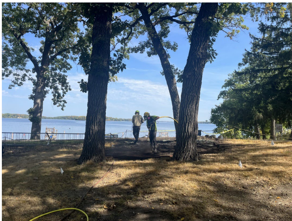
Photograph 8: Air spade work around the oaks on the knoll at The Commons
