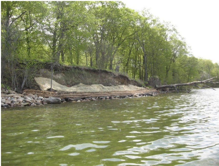
Photo 4 - Post-restoration condition of Big Island shoreline. Photo courtesy of MCWD.
