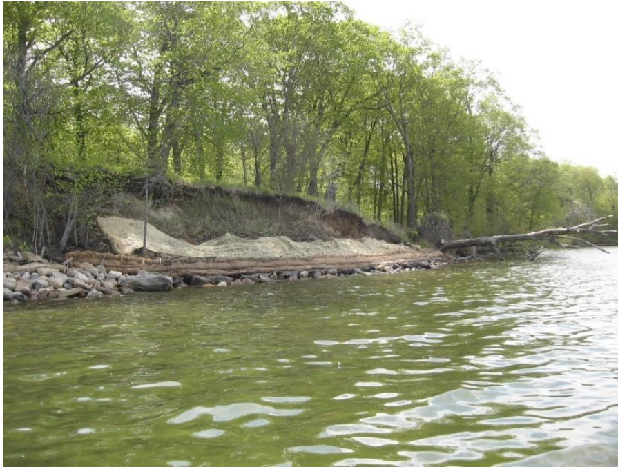
Photo 3 - North face of Big Island pre-restoration. Photo courtesy of MCWD.
